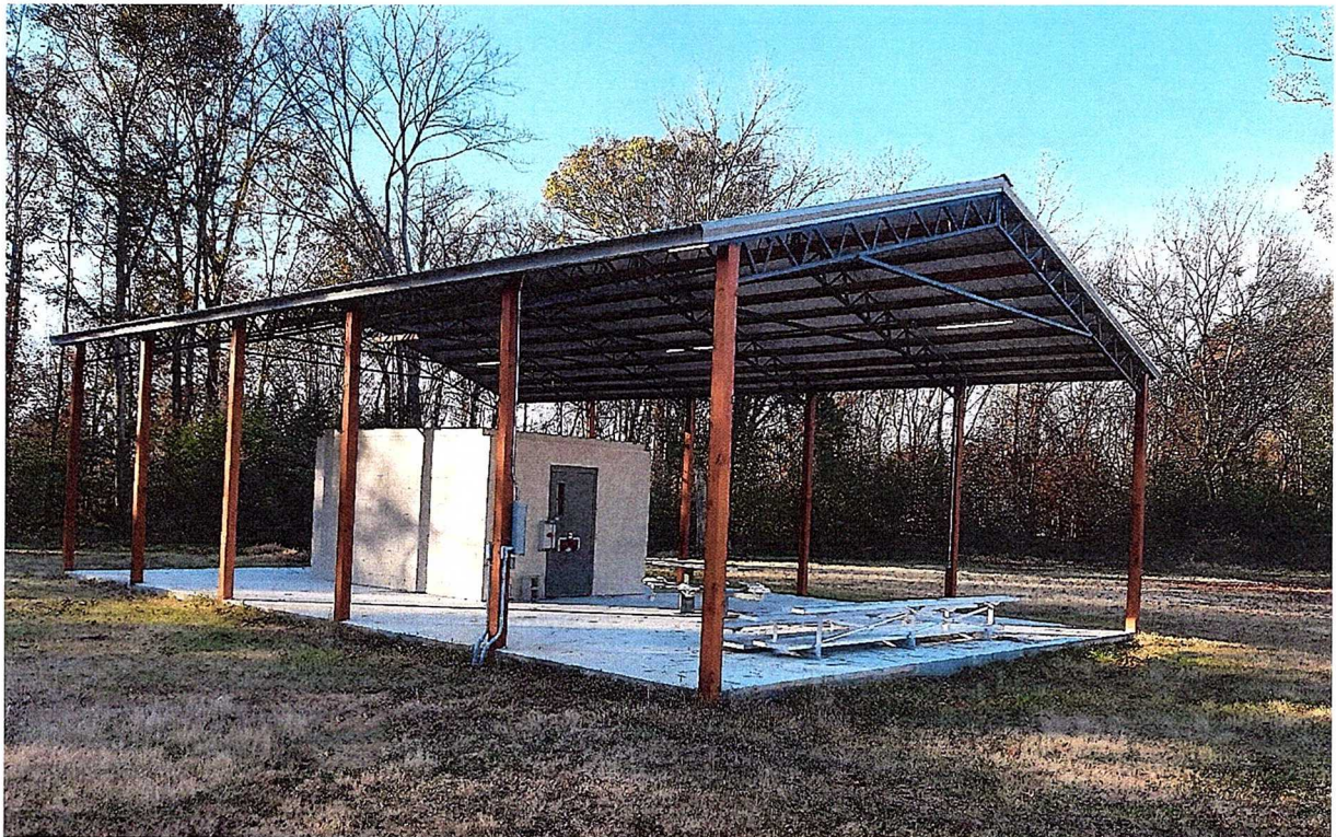
MCSO Correctional Training Facility
