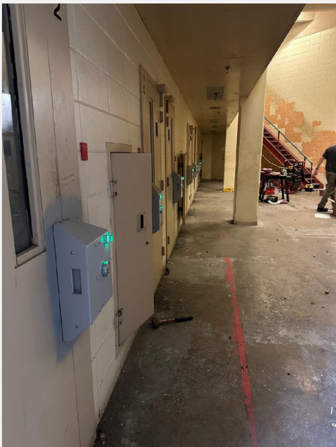
New Willo locks installed
