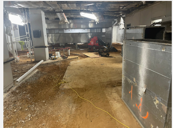
MCDF kitchen renovation.
